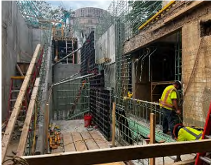
Main Entrance north staircase walls reinforcing steel have now been installed.
