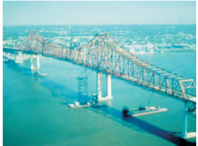
Commodore Barry Bridge 1974
